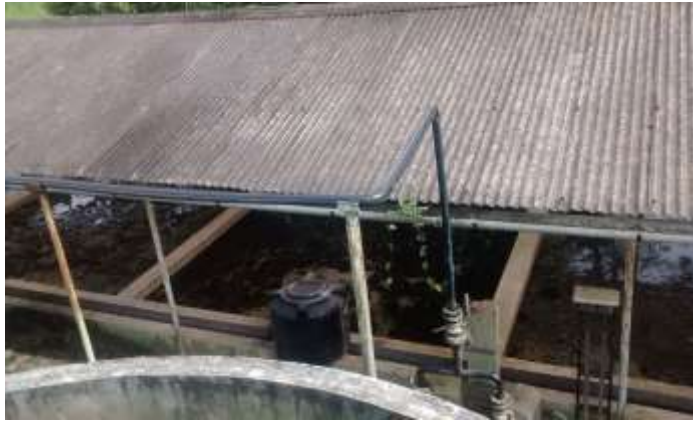
Sludge Drying Bed
