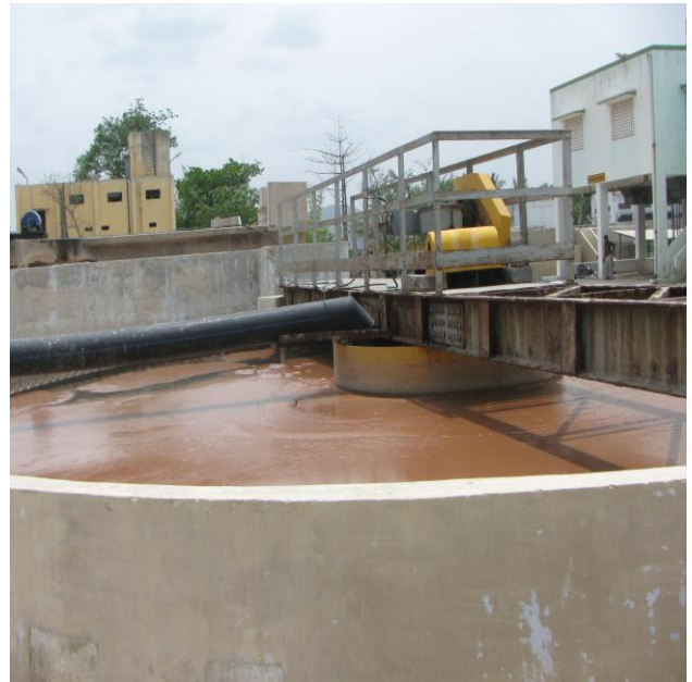
Fig 4: Secondary clarifier
