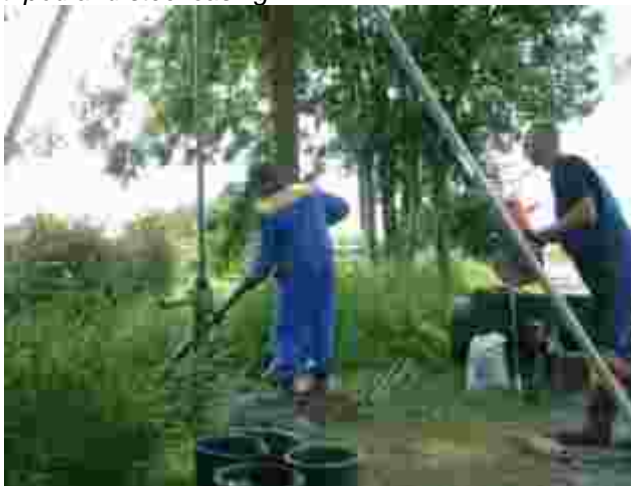
Figure III-2.2-iii.9a Example of hand pulsing, using tripod and steel casing
