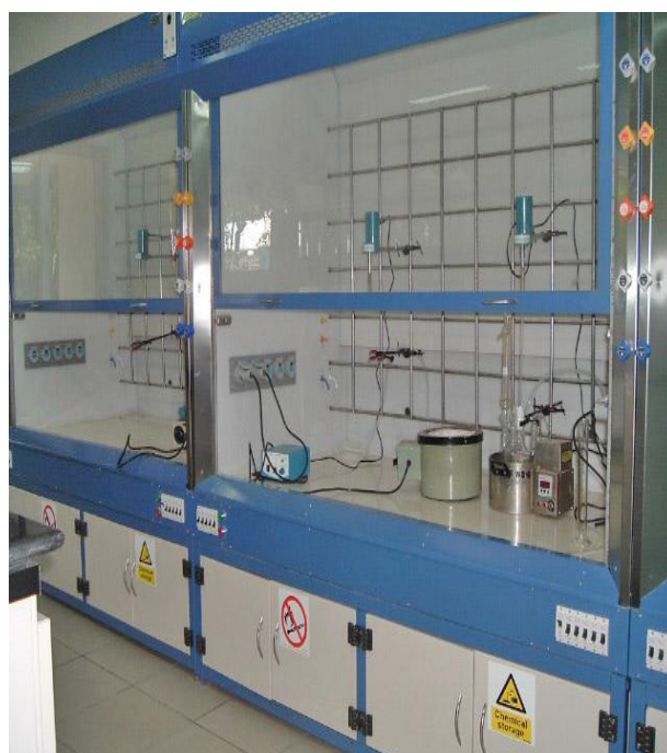
LCV FUME CHAMBERS WITH DIGITAL FLOW METER
