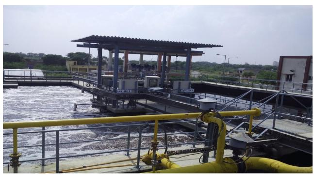
Filtration, aeration, and Nitrification and DO monitoring system
