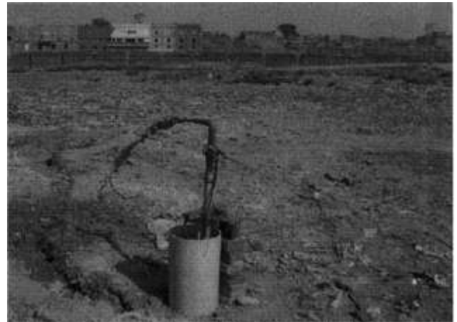
Step vi: Drawing water samples by installation of submersible pump in constructed well
