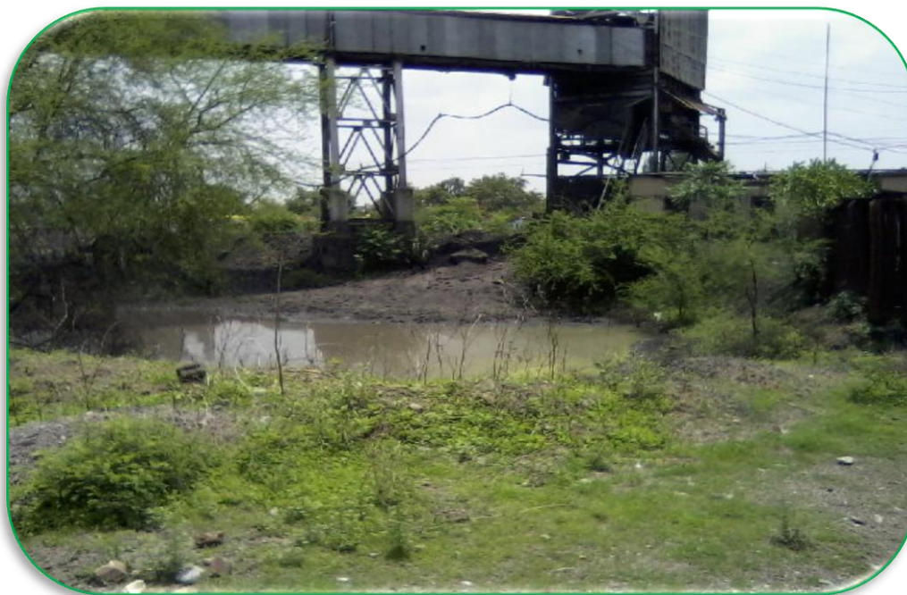
FIGURE 4.17 WATER LOGGED AREA
