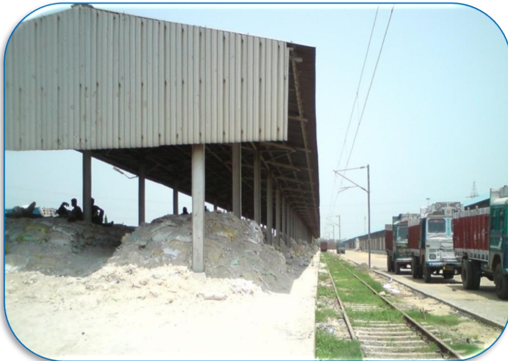
FIGURE 10.4 RESIDUAL WASTE AT SIDING
