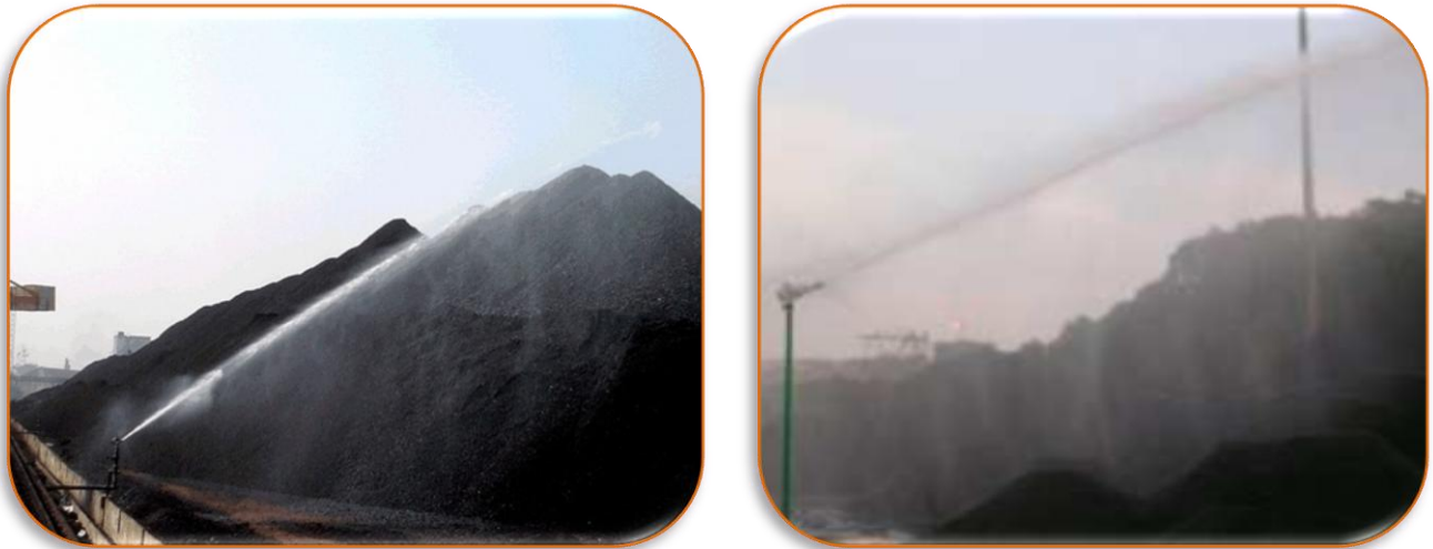
FIGURE 4.24 STOCKPILE WATER SPRINKLER SYSTEM
