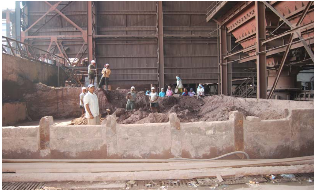
Fig. 5.16: Settled dust being removed from the settling tanks
