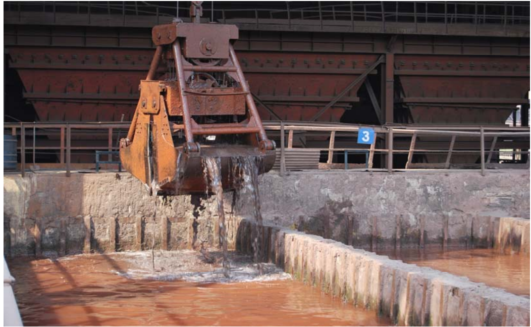
Fig. 5.15: Settled dust being removed from the settling tanks
