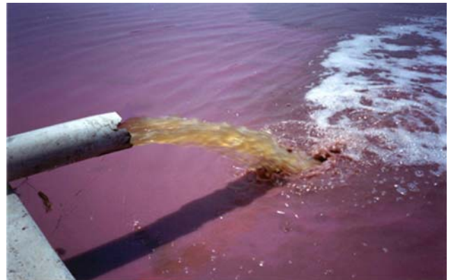
SUPERNATANT FROM SETTLING TANK
