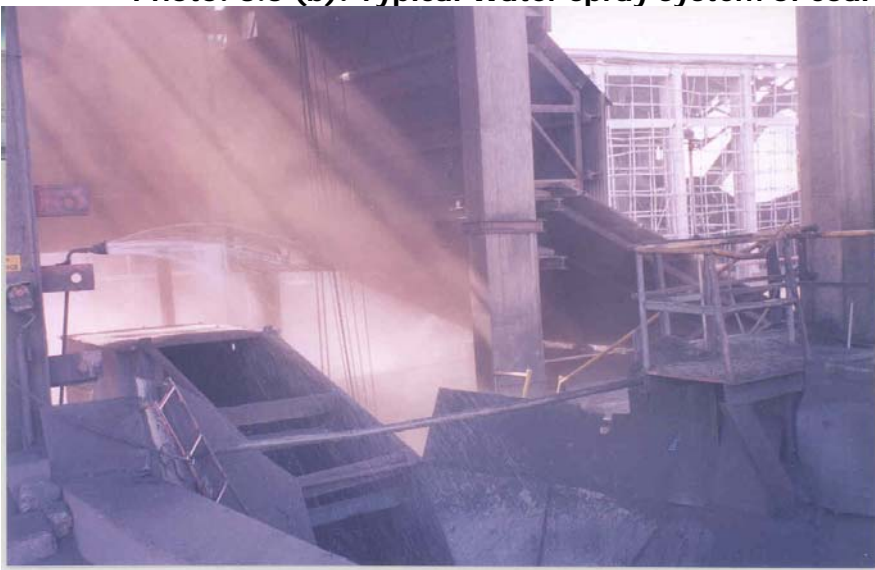
Photo: 3.5 (b): Typical Water spray system of coal dump hopper
