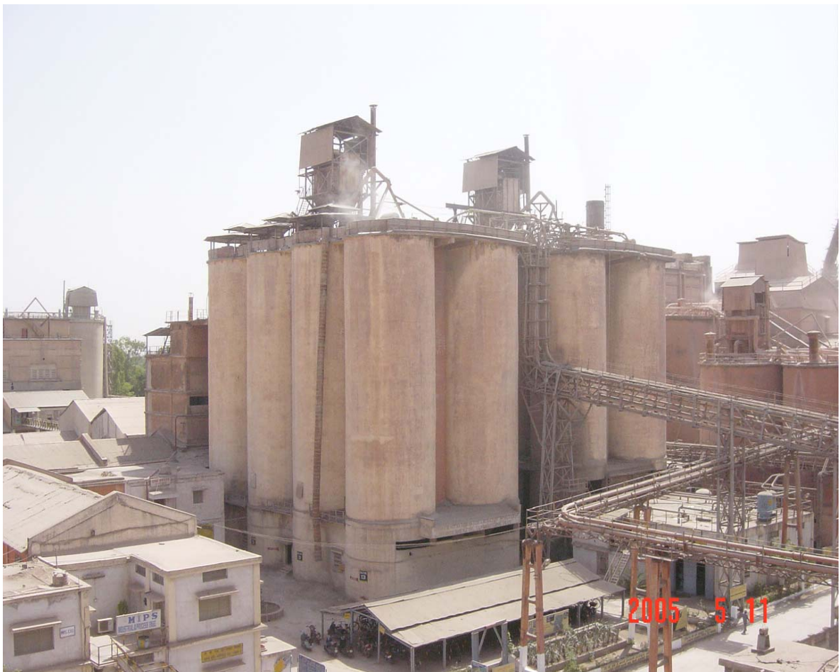
Photo 3.7: Typical Fugitive Emissions from Cement Silo Tops
