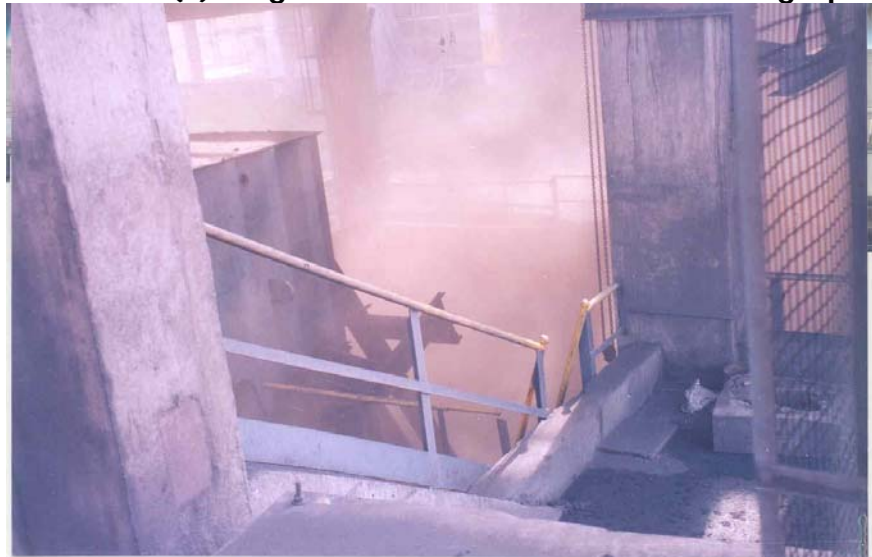
Photo: 3.5 (b): Typical Water spray system of coal dump hopper
