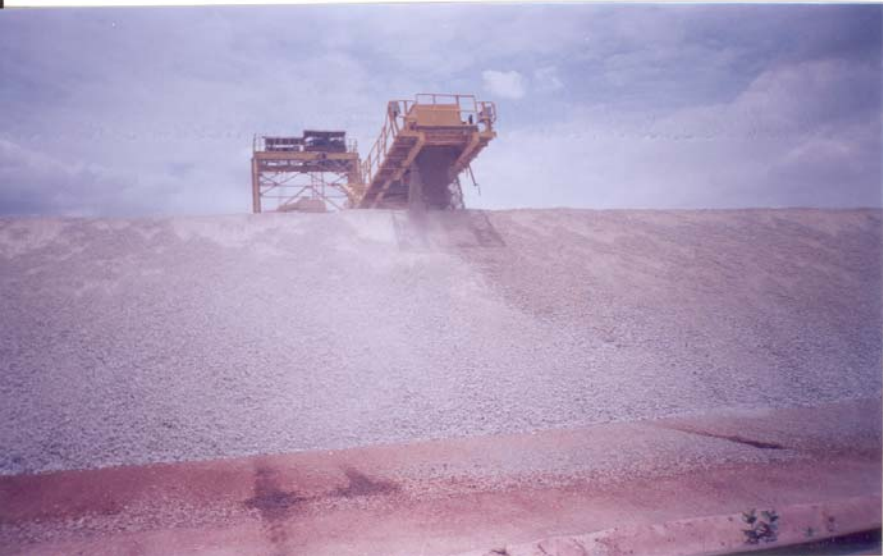
Photo 3.3: Views of various Limestone Storage arrangements
