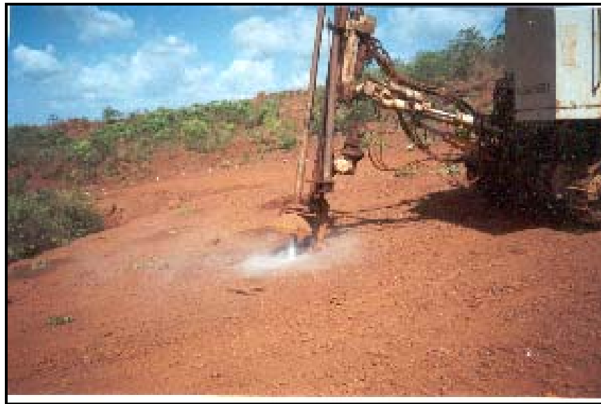
Fig. No. 5.1.1.2 Wet Drilling in Operation
