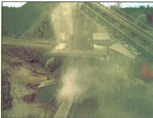
Without Dust Control
