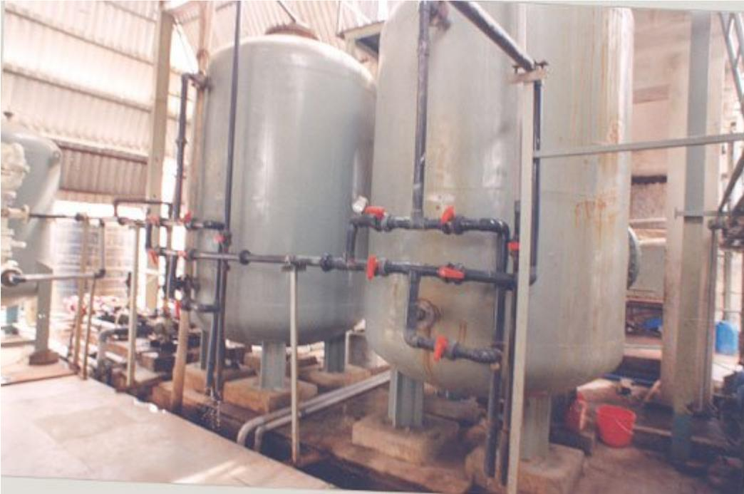
**Activated Carbon Adsorption Plant**
