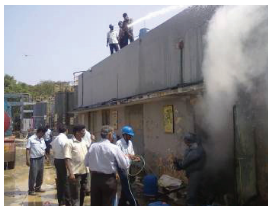
Figure 14.7 : Bromine Gas Leakage at pharmaceutical unit in Cuddalore, Tamilnadu
