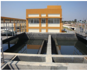
Equalization tanks
