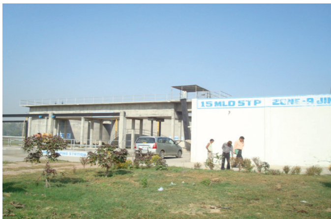
Figure 14.1 : 15 MLD Sewage Treatment Plant at Jind
