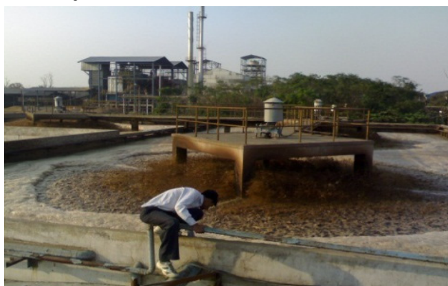
Figure 10.3 : Clarifier-cum-aeration System
