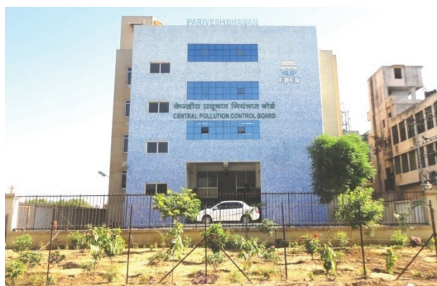
Figure 14.15 : CPCB Zonal Office-cum-Laboratory Building at Vadodara
