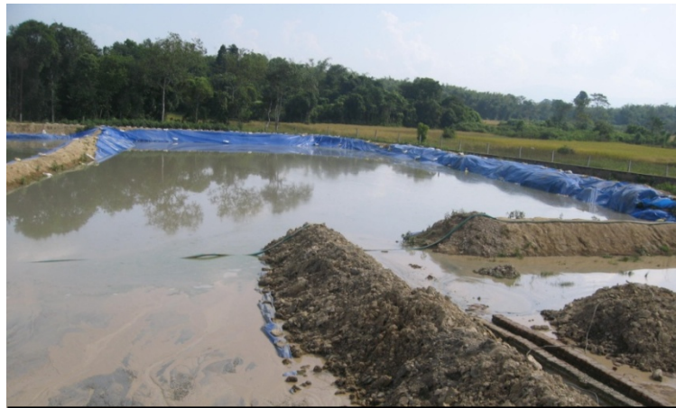
Drill cuttings and drill muds are not properly managed in the drill sites
