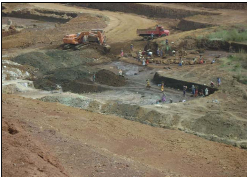
Chrome ore is being lifted from Seam at the bottom of the pit
