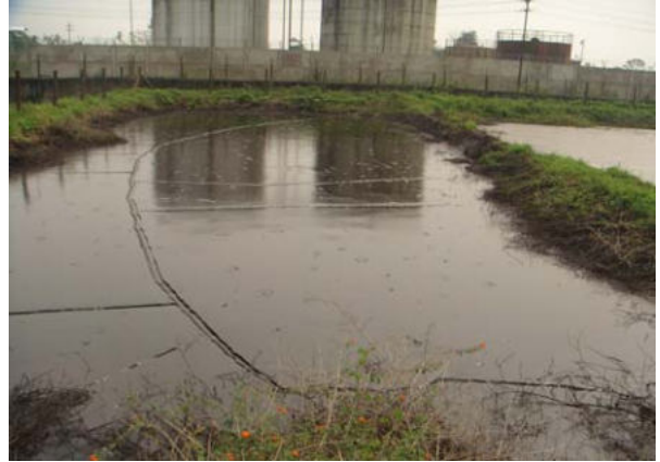
Sludge pit inside the Kathalguri Mud Preparation Station
