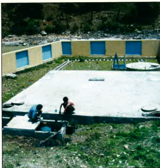
Septic tanks on the bank of river Bhagirathi at Tekhala
