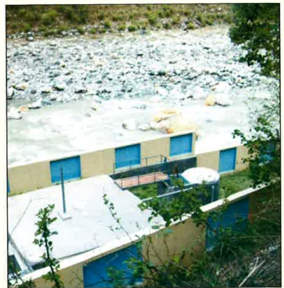
Septic tanks on the bank of river Bhagirathi at Gangotri
