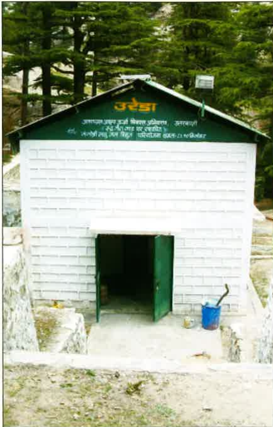
Ureda Hydroelectric projects on tributary of river Bhagirathi
