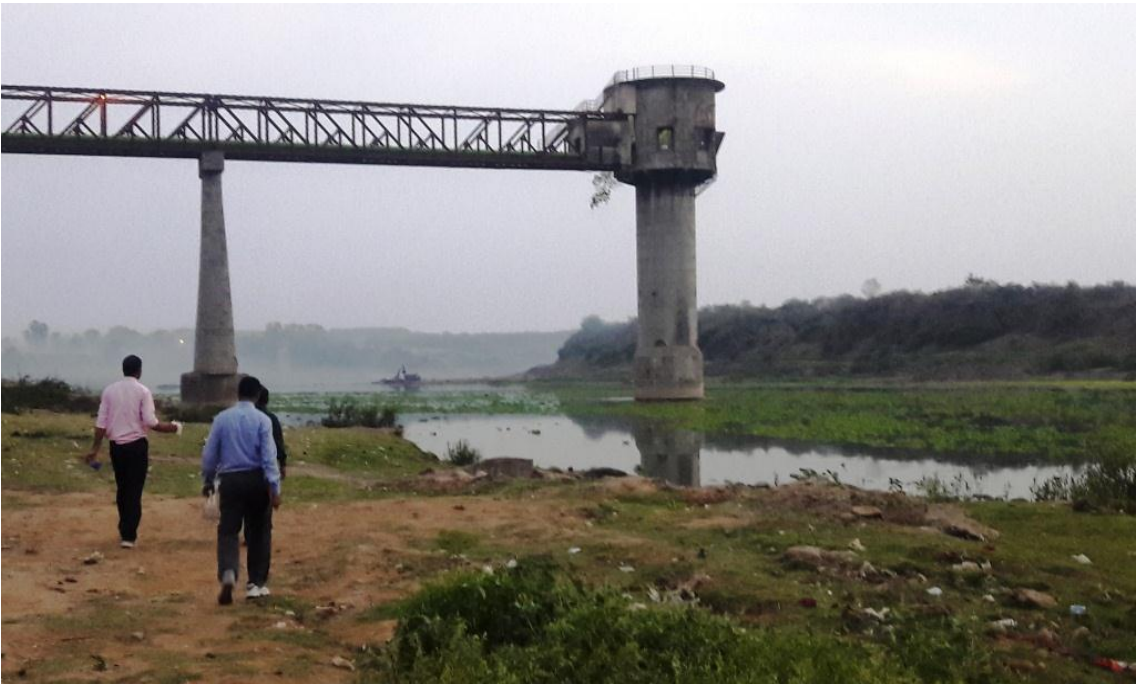
Photographs-9 & 10: SWQM location-5
