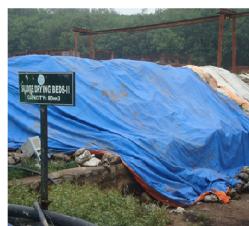
Hazardous waste stored in open space
