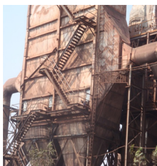
ESP Installed to Control SPM
