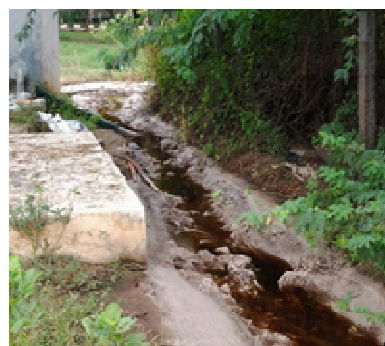
Discharge of treated effluent into drain
