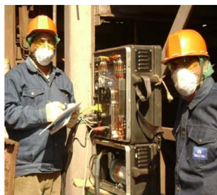
Source Emissions Monitoring
