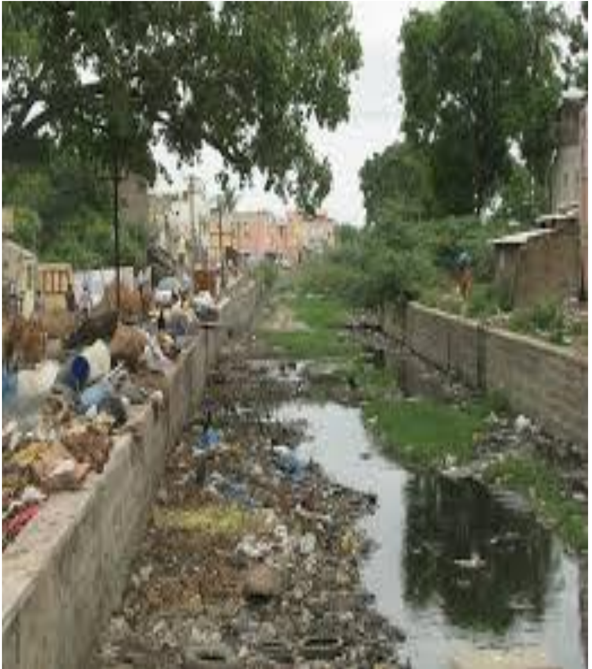
Figure 6.1: Indiscriminate dumping of C & D waste results in choking drains
