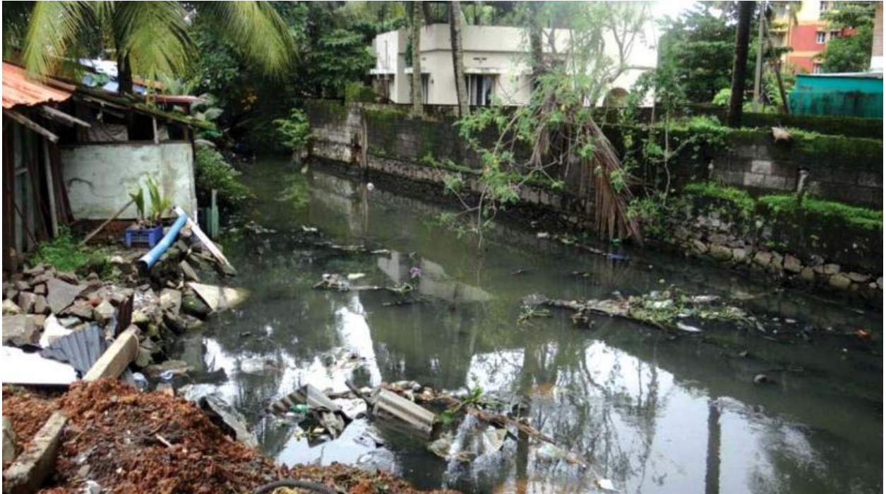
Figure 7.1: Dumping of C & D wastes clogs drains in cities
