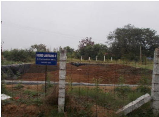
Secured land fills site
