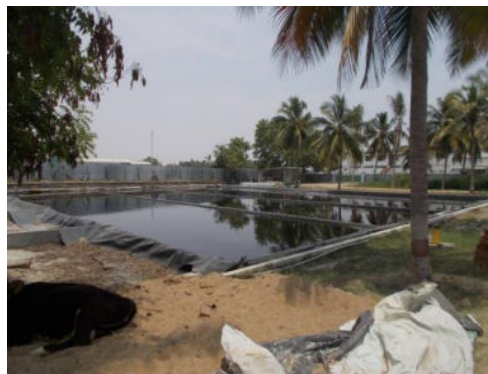
Solar Evaporation ponds with concentrated effluent
