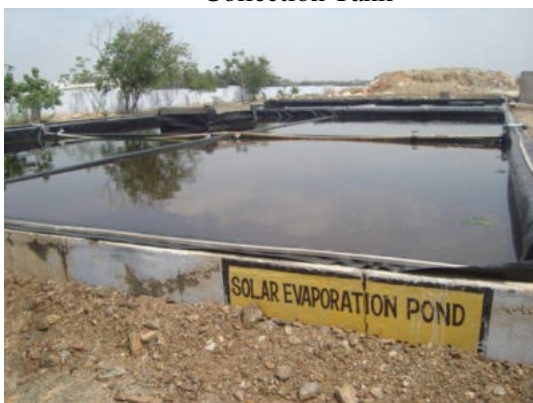
Solar Evaporation Pond
