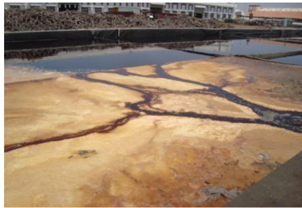
Accumulated salt in solar evaporation
