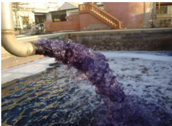
Effluent Receiving tank
