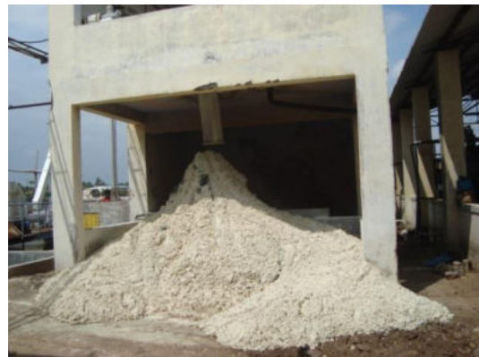
Chemical sludge dewatered in filter press
