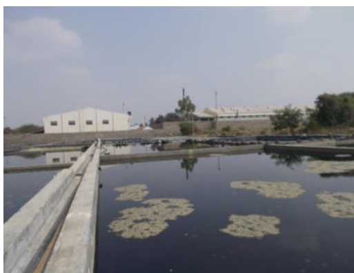
Accumulated mother liquor in solar evaporation pond
