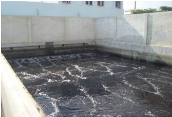
Homogenization tank
