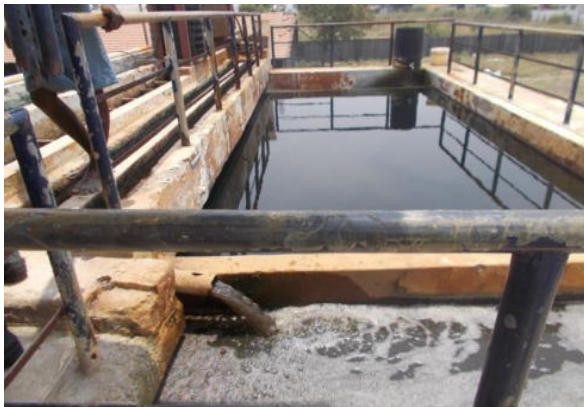
Poor house keeping in Effluent collection system and in RO system
