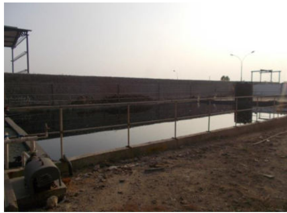
MEE with 3 effect forced circulation system Solar ponds for natural evaporation of concentrated effluent
