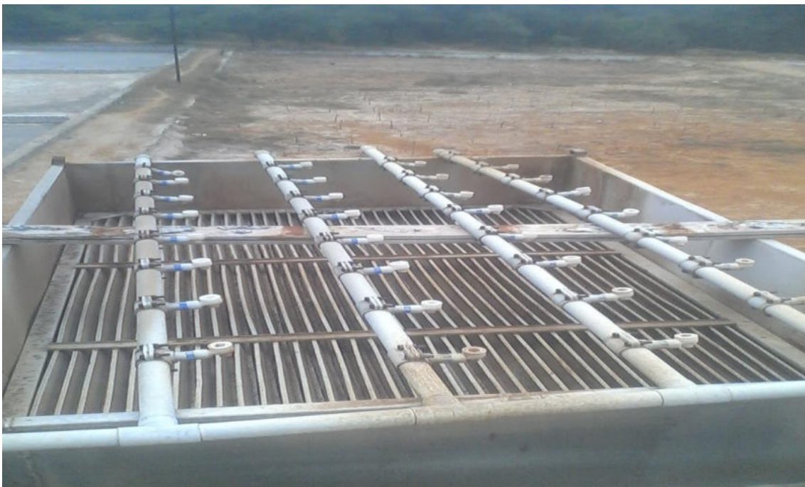
Fig: 3.6 Demister Configurations
