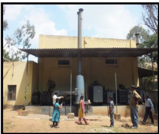
Chimney connected to hood system with water scrubber
