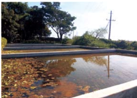
Solar Evaporation Pond
