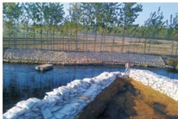
Green Bridge Technology at BudhaNala, Ludhiana
