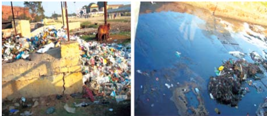
Choked drains by Solid waste
