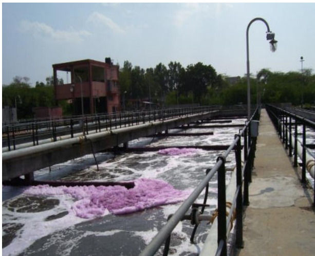
Colored effluent in aeration tank
