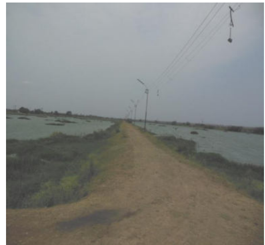
Treated water collection ponds
