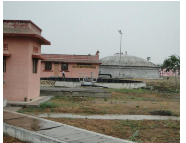
view of sludge digester
