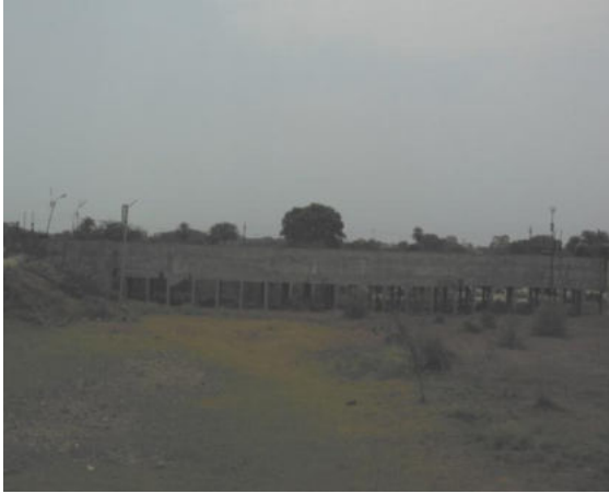
Raw Sewage Collection Tank
