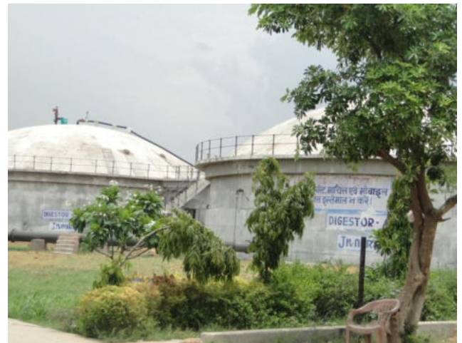
view sludge digesters
