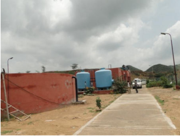
Cemented road in the premises
