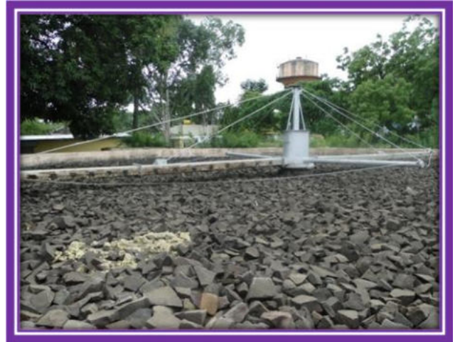
Trickling Filter
