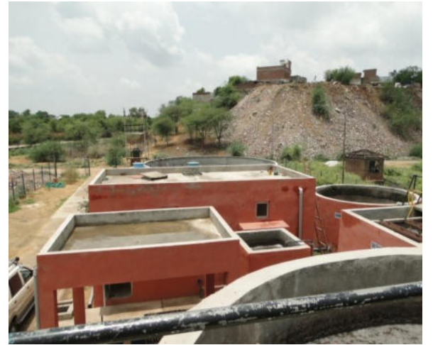
View of STP structures
