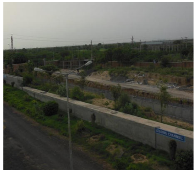
Construction of New 50 MLD Plant
