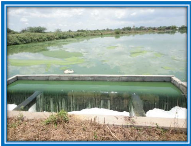
Waste Stabilization Pond overflow
