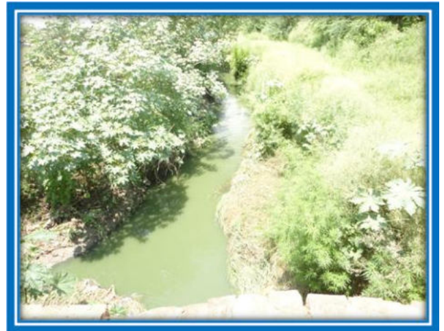
Treated water outlet
