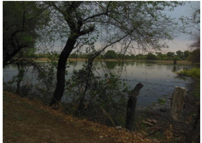
Treated water storage lagoon
