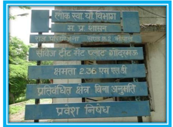
Gondarmau STP Primary treatment unit
