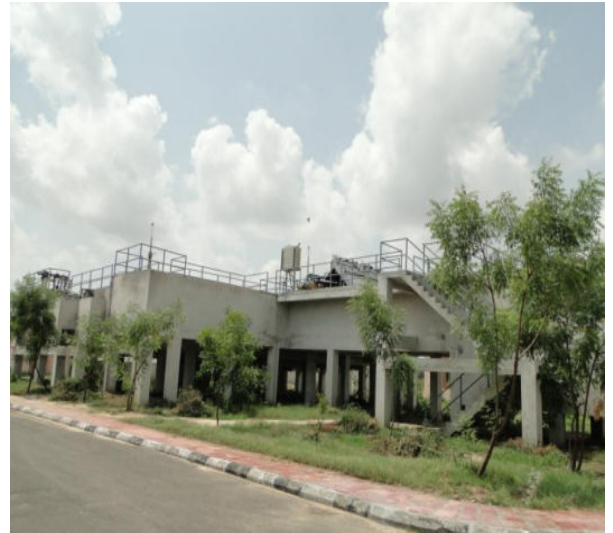
view of STP
