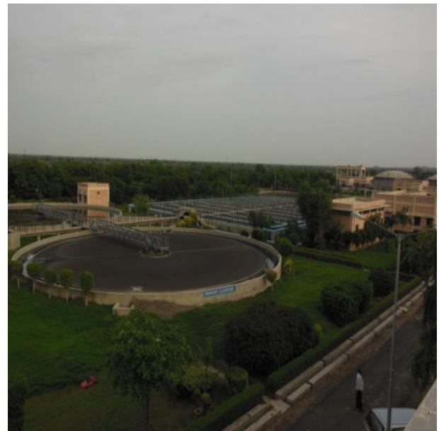
View of primary Clarifier
