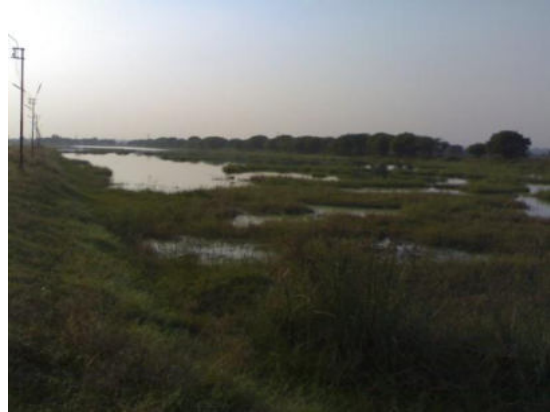
Waste stabilization pond at Sadawal village, Ujjain
