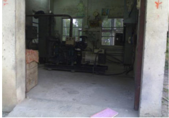
Pump house for sewage pumping at KT plant
