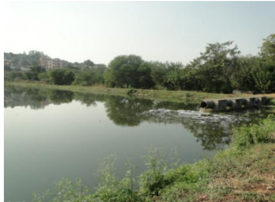
Inlet of Oxidation Pond
