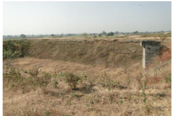
Unused Oxidation Pond
