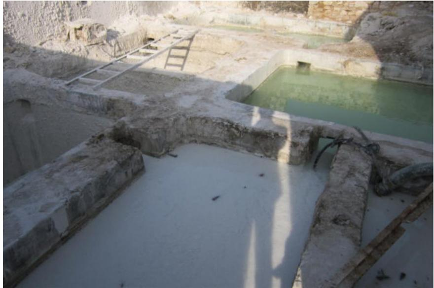
process, make slurry along with the water, spread over the block. To recycle the water & to settle the marble dust, zigzag water-cum-dust storage tank are constructed. Through this zigzag movement & sedimentation process the dust settled at bottom. Alum as coagulator can enhance this sedimentation rate. The supernatant is again recycled to gang saw. In this settling process average water loss is upto 1000-1500 Ltrs per day. The semi-solid marble
