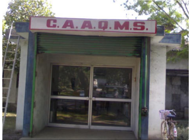
CAAQMS at Ambuja Cement
