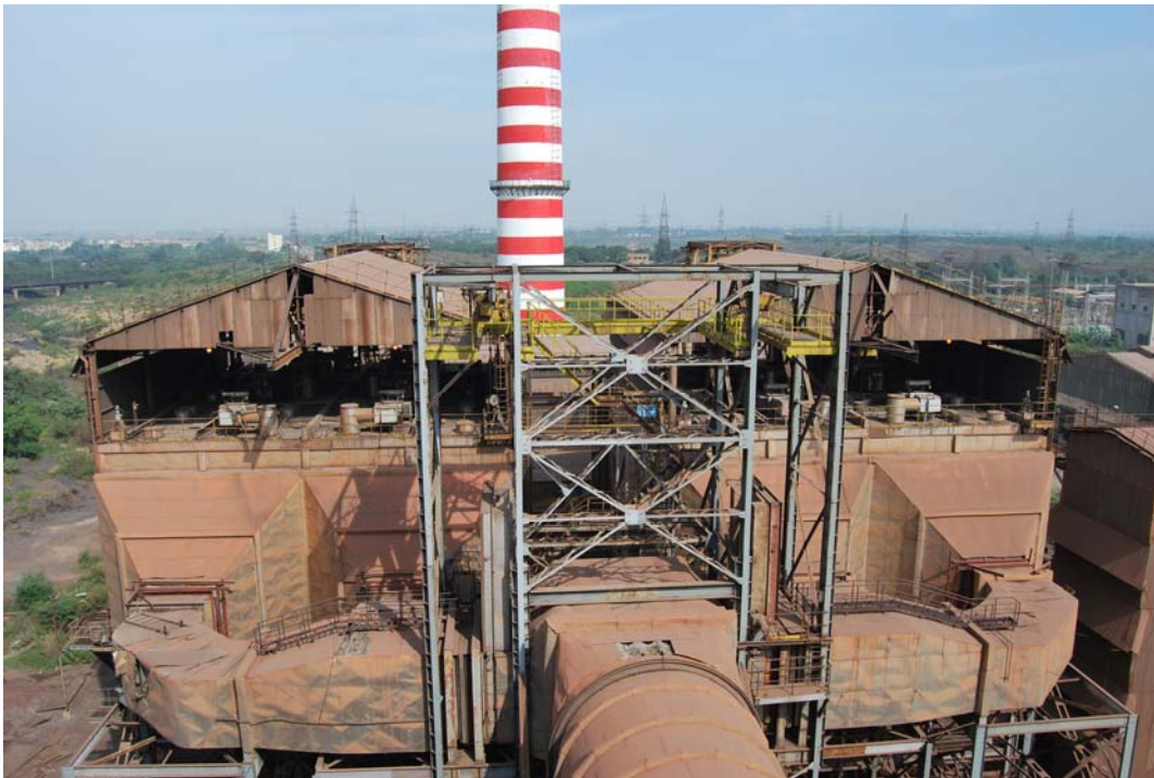
Fig. 3.14: Process gas de-dusting ESP with stack
