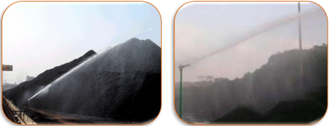
FIGURE 4.24 STOCKPILE WATER SPRINKLER SYSTEM
