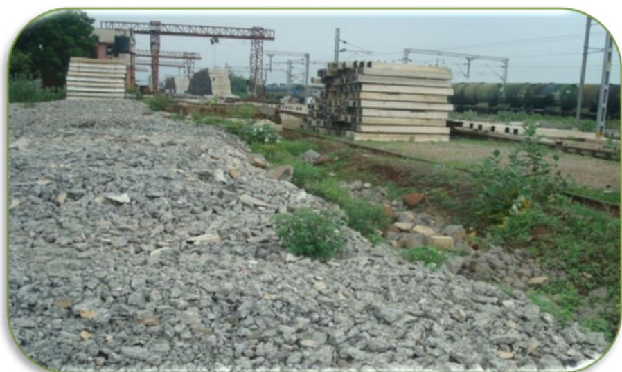
FIGURE 9.3 WASTE MATERIAL AT RAILWAY SIDINGS
