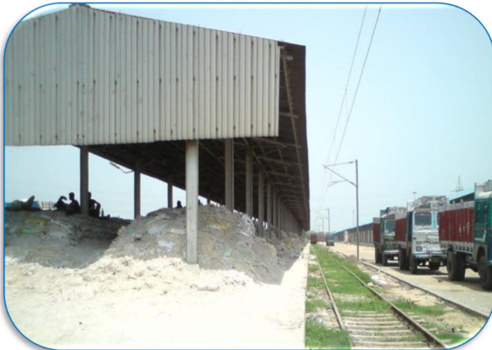
FIGURE 10.4 RESIDUAL WASTE AT SIDING
