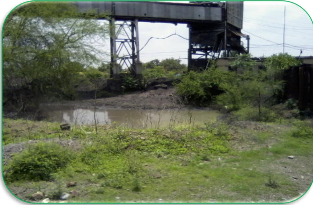
FIGURE 4.17 WATER LOGGED AREA
