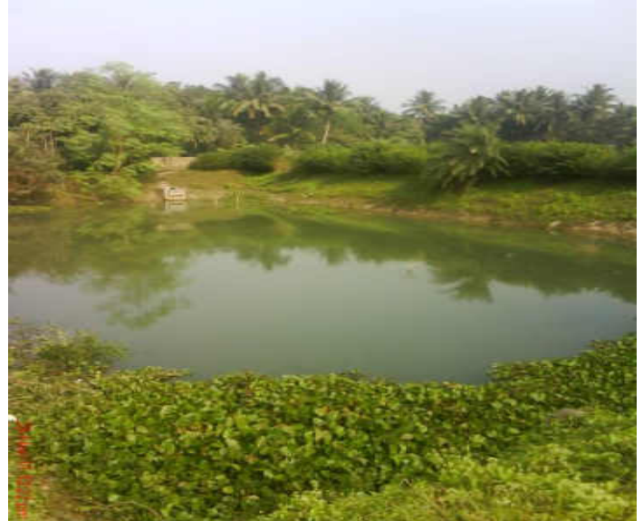
Picture 21: STP at Barrackpore
