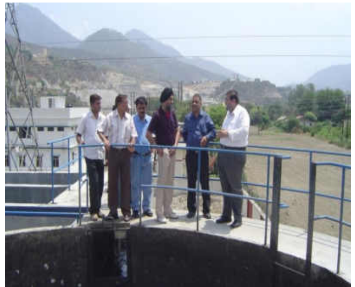
Picture 15: STP at Sringar
