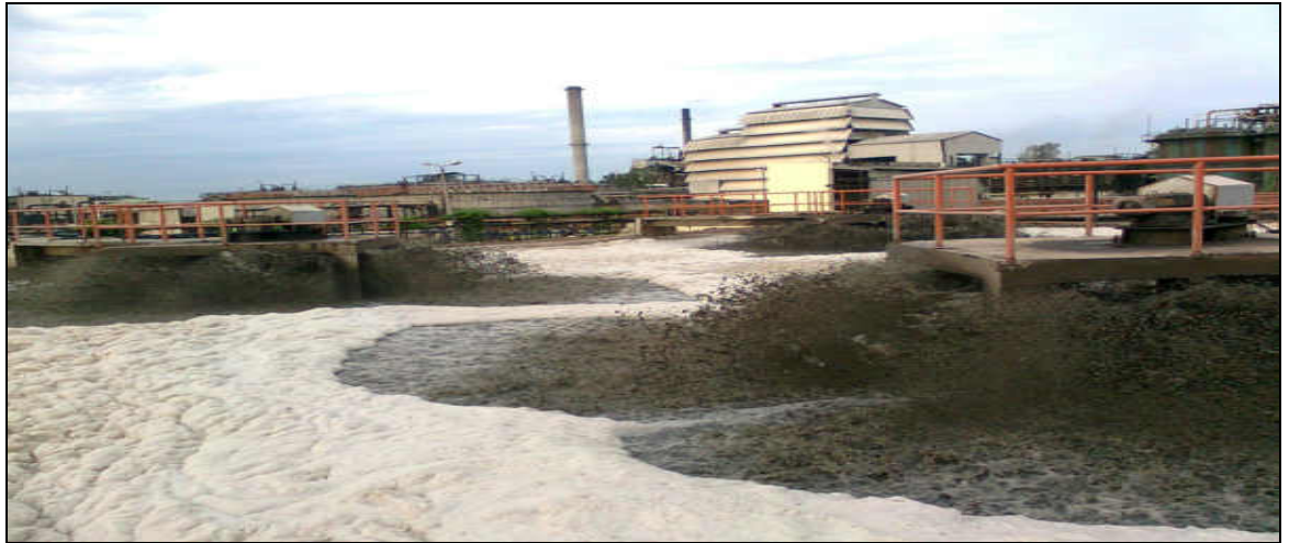
Pic.6: Aeration tank of Chandigarh Distillery
