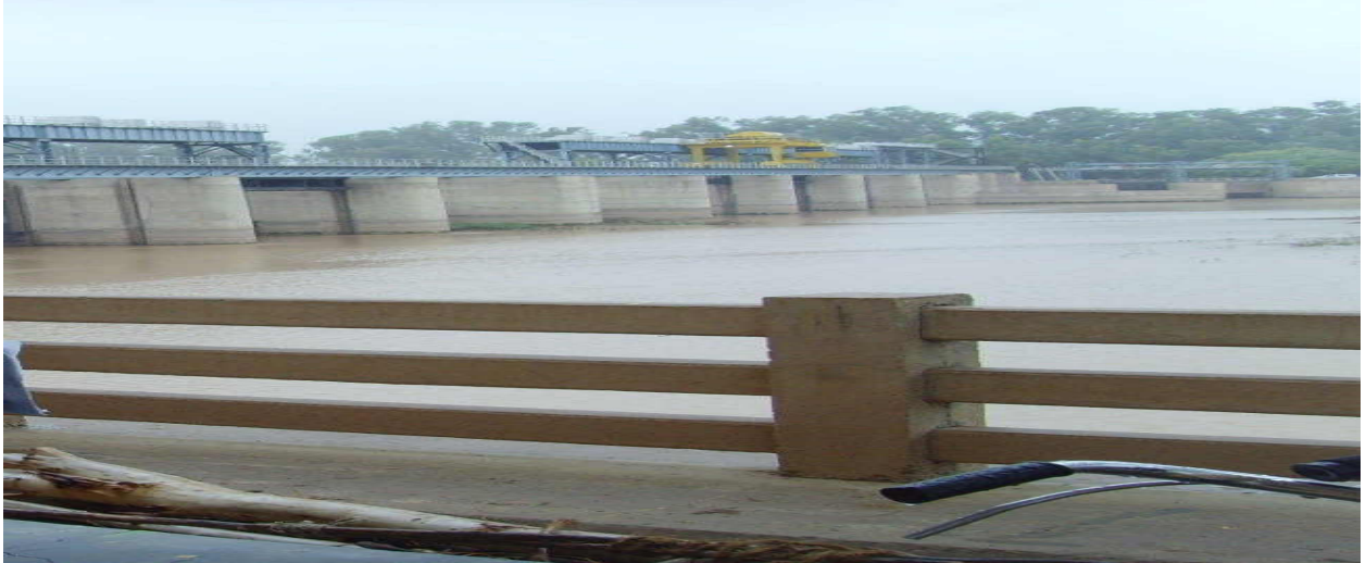
Pic.13: River Ghaggar at Ottu Weir
