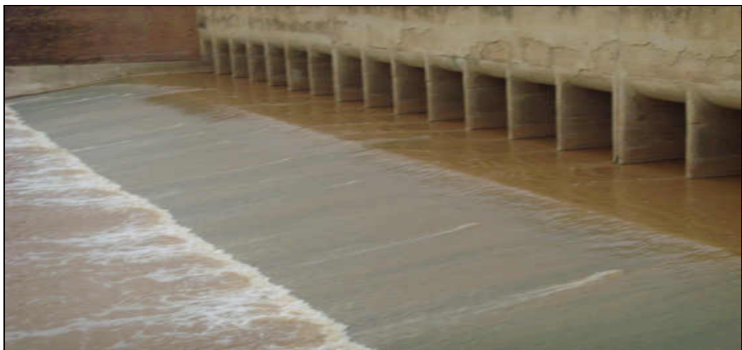
Pic. 12: River Ghaggar at Chandrapur Siphon, Haryana
