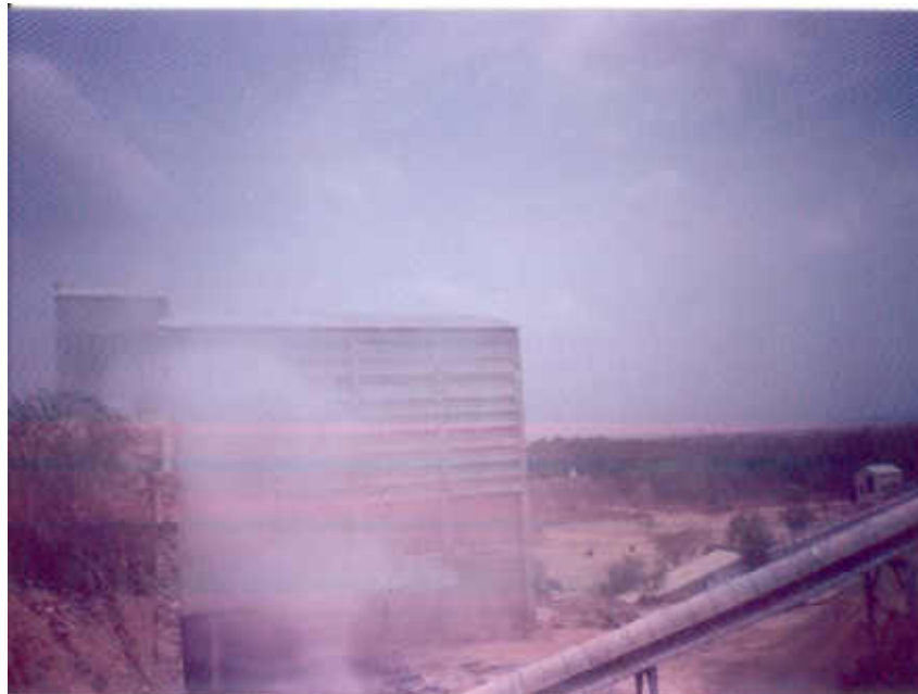
Photo 3.2: Emission from Lime Stone Crusher House
