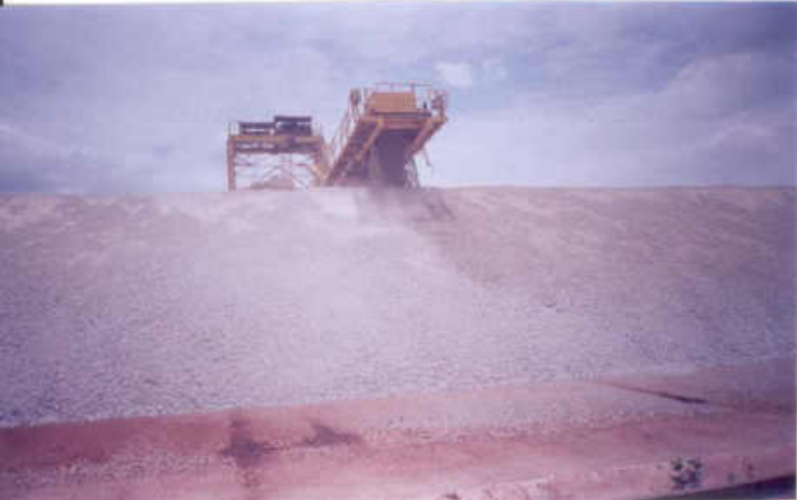
Photo 3.3: Views of various Limestone Storage arrangements
