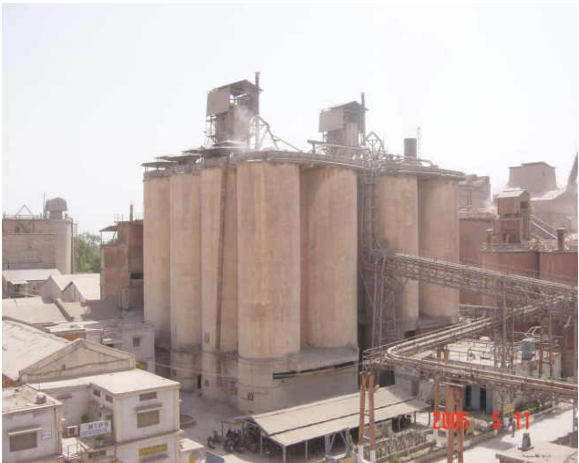
Photo 3.7: Typical Fugitive Emissions from Cement Silo Tops
