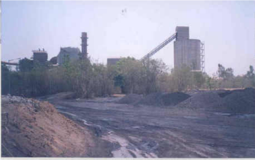
Photograph 3.8: Coal outdoor storage
