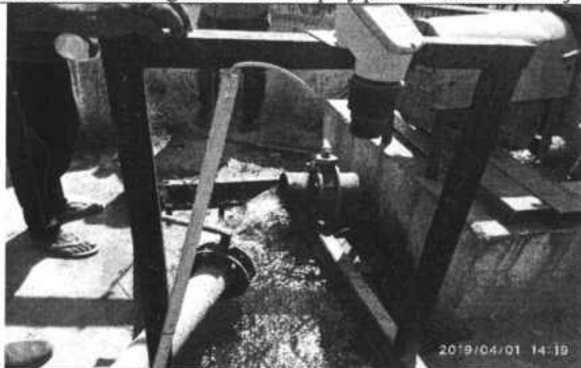
Fig.5: Arrangement for bypassing tertiary treatment
