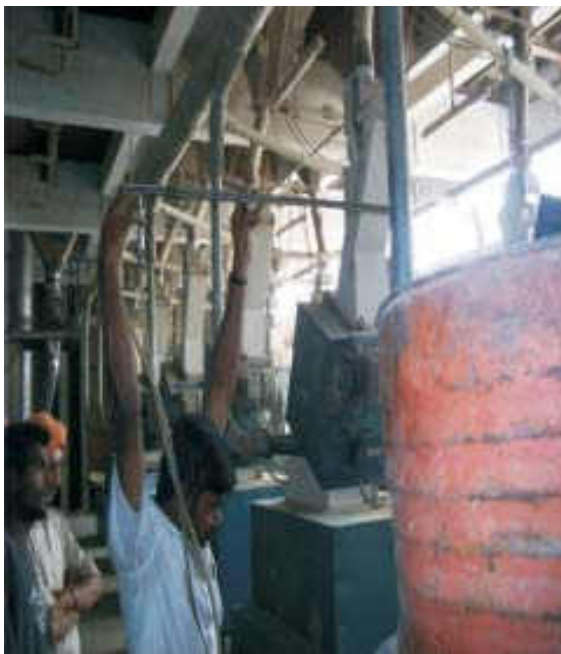
Fig.6.9. Outlet from Single Huller (Port Hole 4) on 3 rd floor
