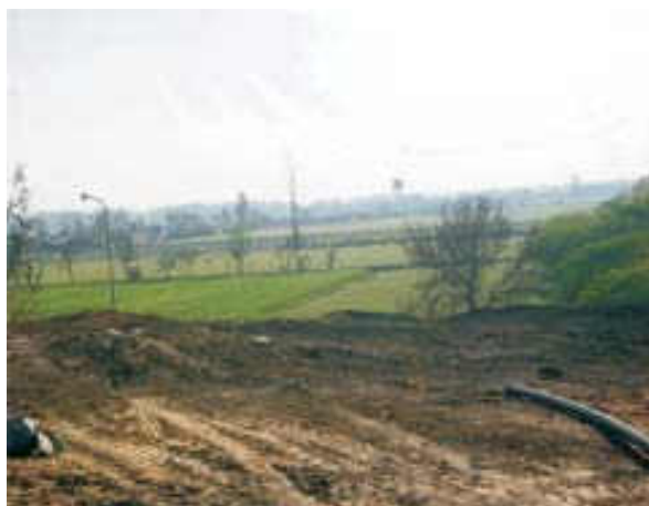
Fig 4.18-Layer of soil after disposal of boiler ash
