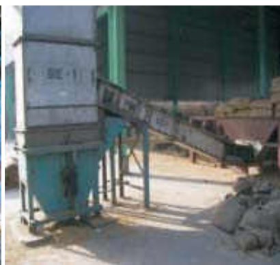
Fig 5.2(a)-Bucket Elevator Fig 5.2(b) Conveyer
