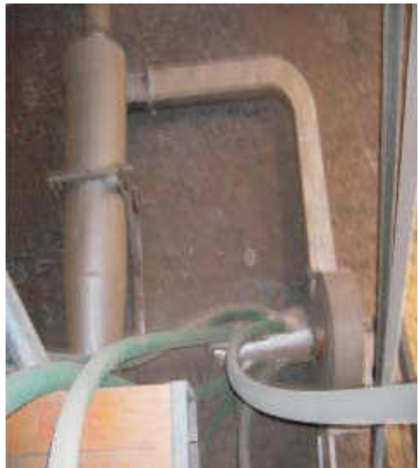
Fig 5.18-Variou flexible suction pipes sucking from various equipments and passed through a common cyclone in small rice mills
