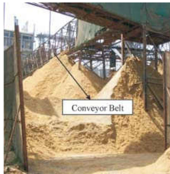
Fig 4.5-Rice husk conveyance in storage yard using conveyor belts Conveyor Belt
