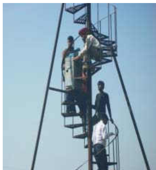
Fig.6.14 Near ETP Plant
