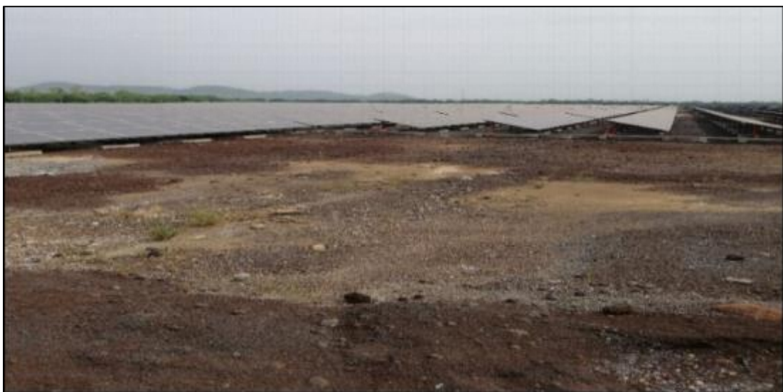
Figure 9: Solar panels on top of the capped Jarosite ponds no. 1 and 2 at Debari
