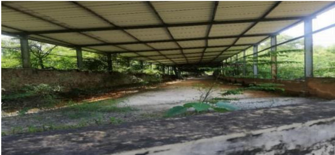
Figure 15: Covered pathway for dumpers carrying stabilized Jarosite at EDL
