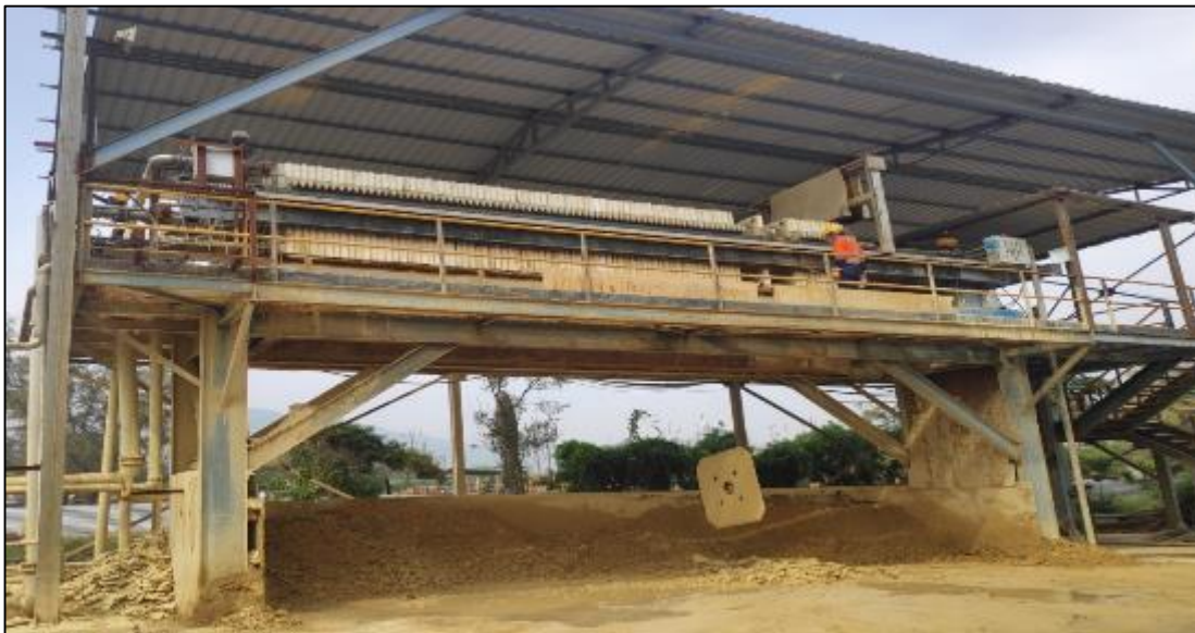
Figure 8: Filtered Jarosite before dispatch to cement plant at Debari unit
