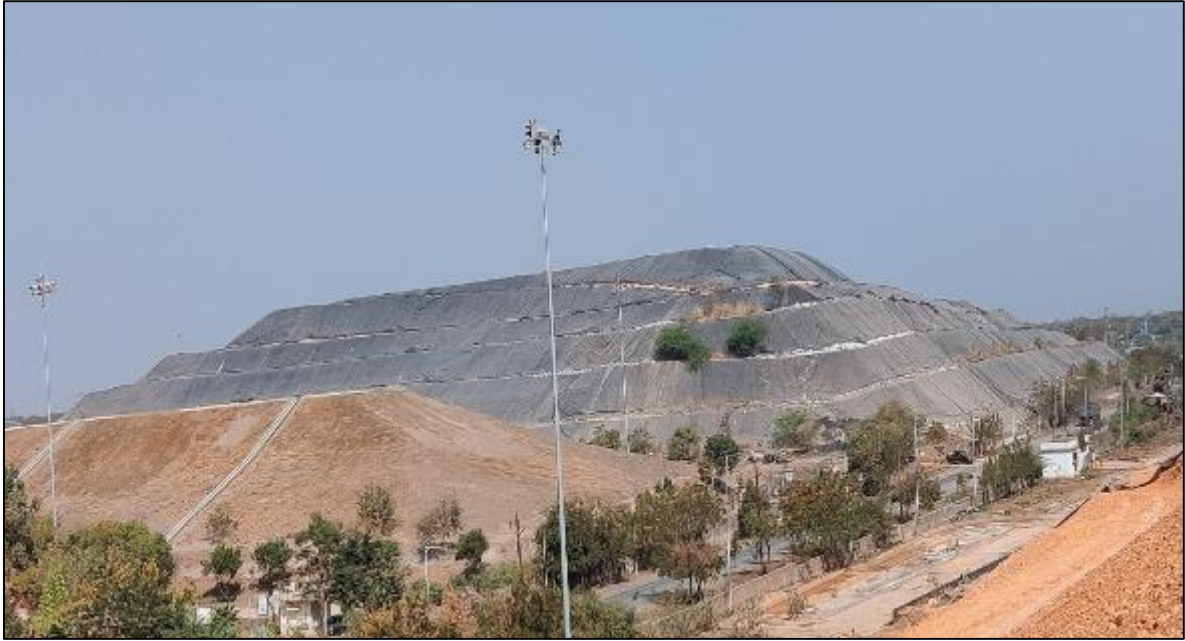
Figure 32: Old stabilized Jarosite Pond at Dariba (Phase 1 and Phase 2 exhausted and covered with HDPE)
