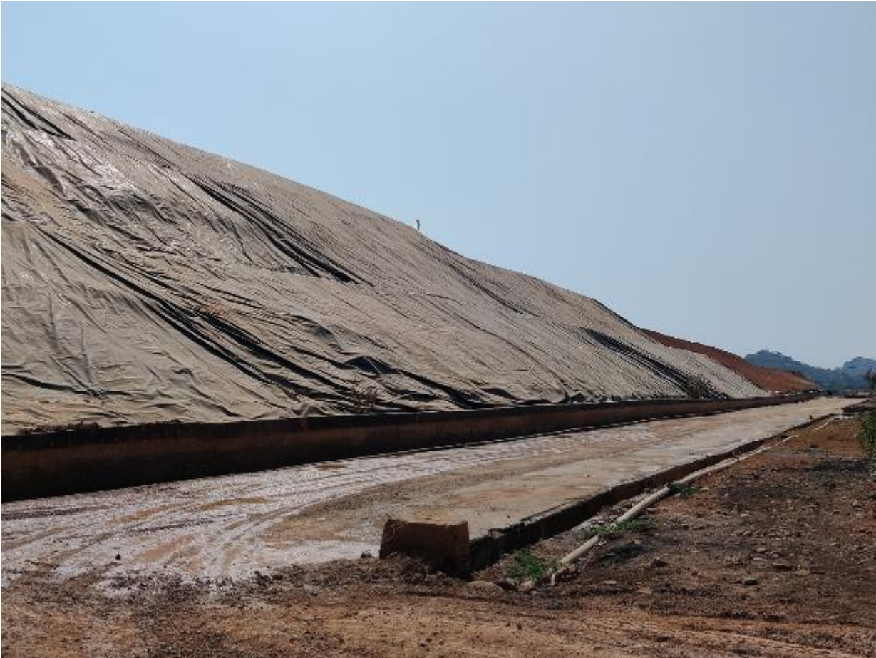
Figure 33: Active Pond at Dariba (Phase 1 exhausted and covered with HDPE; Phase 2 is operational)
