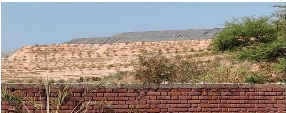
Figure 26: Plantation (carried out by TERI) on a section of Old Stabilized Jarosite pond 2 at Chanderiya unit
