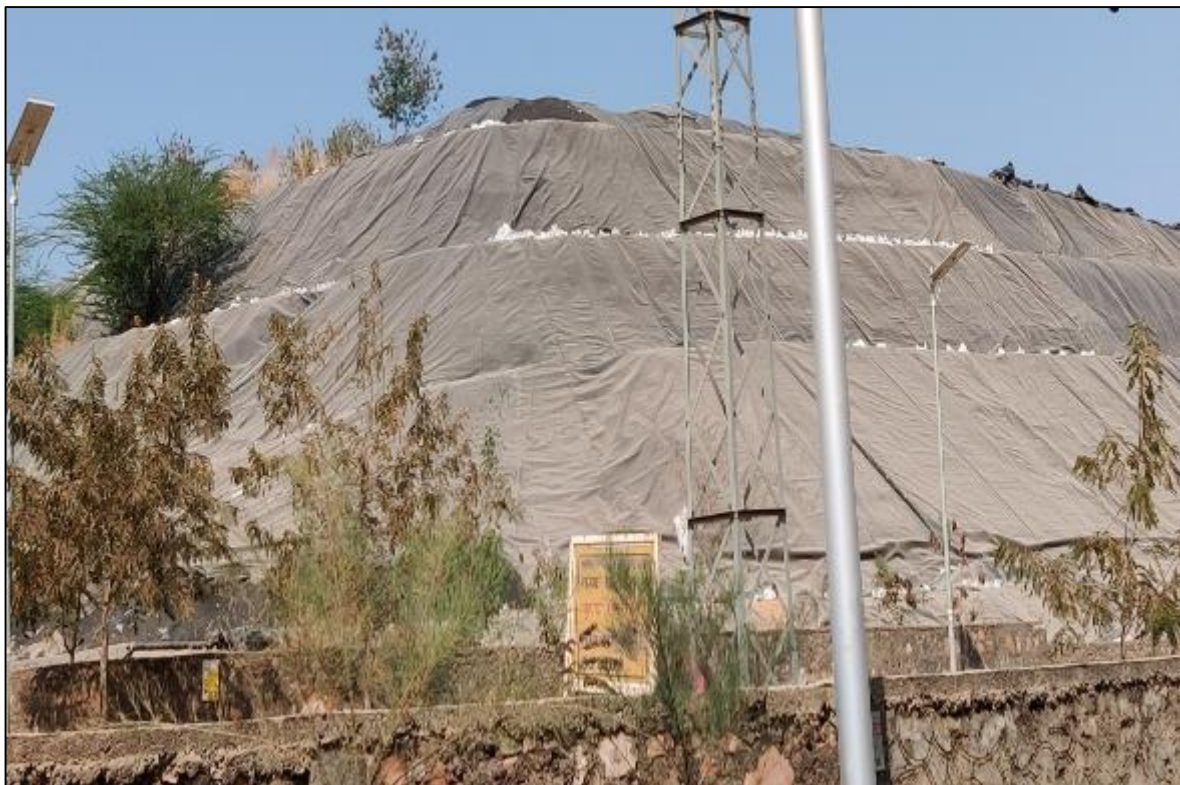
Figure 31: Old stabilized Jarosite Pond at Dariba (exhausted and covered with HDPE)
