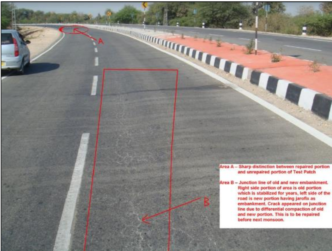
Figure 28: 300 m test patch of road constructed using stabilized Jarosite
