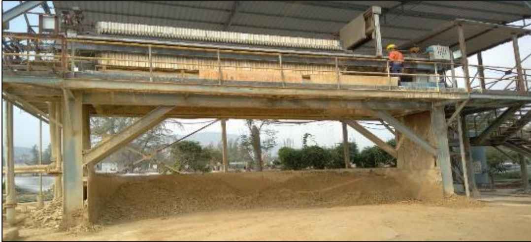
Figure 7: Filter Press at Debari Unit
