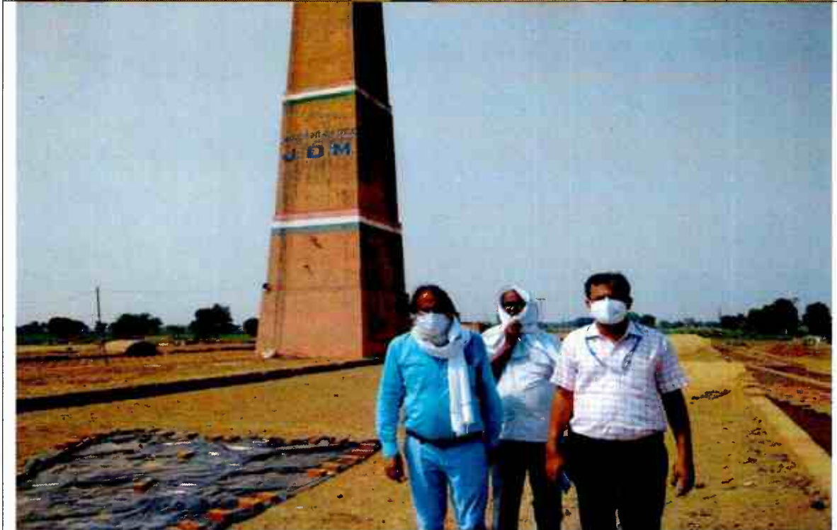
Zig-Zag type Brick Kiln with induced draft at Chhaata, Mathura.
