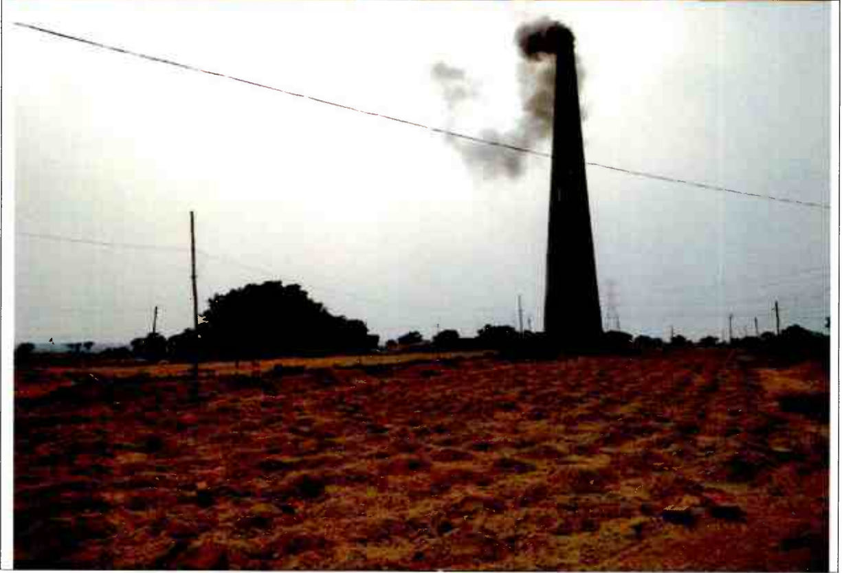
Black fumes from the stack of Brick Kiln unit located at Maant, Mathura.
