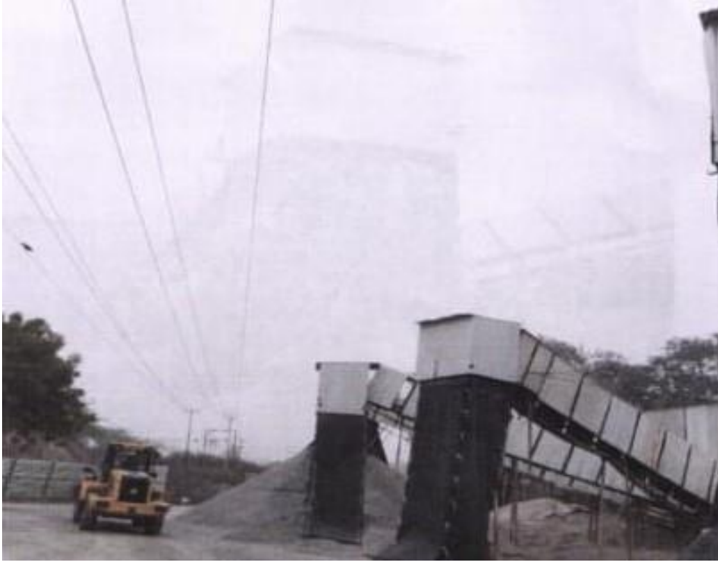
Figure-2(a): Chute from top of discharge point
