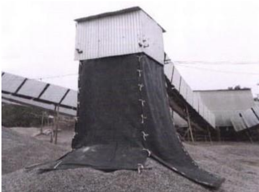
Figure-2: Chute from top of discharge point
