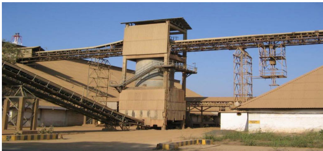
FIG. 2. Phosphate rock silo & conveyance system
