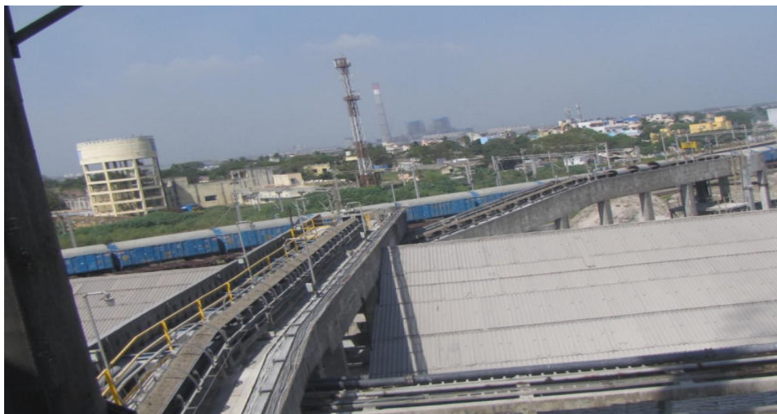
FIG. 4. Conveyance of phosphogypsum to the Stack Area through 'Belt Conveyor'
