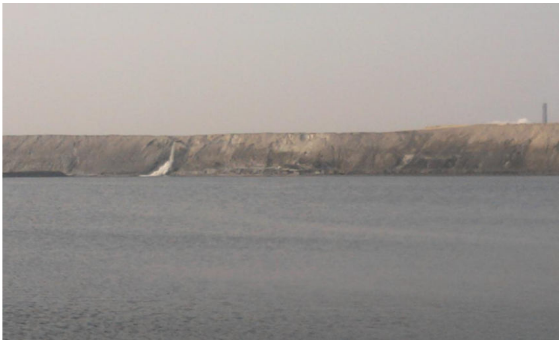
FIG. 9. Cooling water collection in 'surge pond' over the phosphogypsum stack
