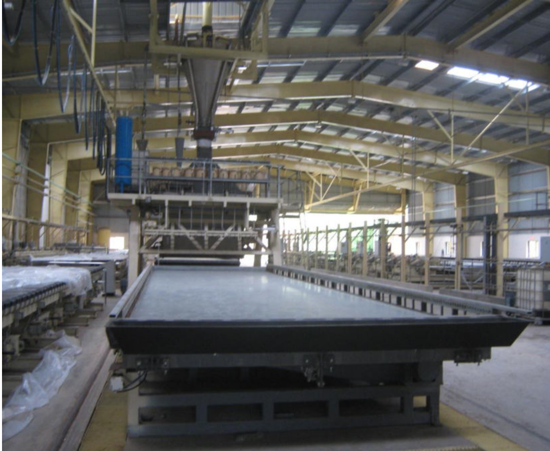
FIG. 12. Plant & Machinery for plaster board/panel manufacturing using phosphogypsum
