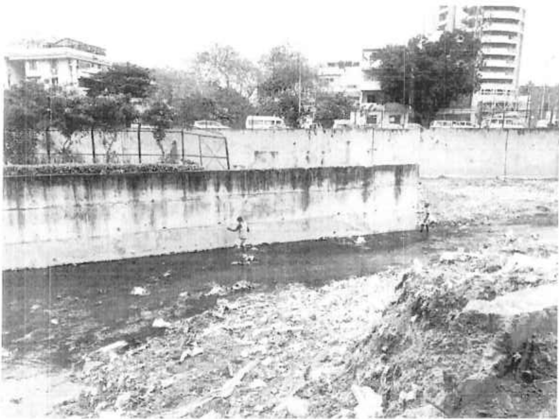
Figure 1: Flow measurement at storm water drain C-100 downstream of Ulsoor Lake
