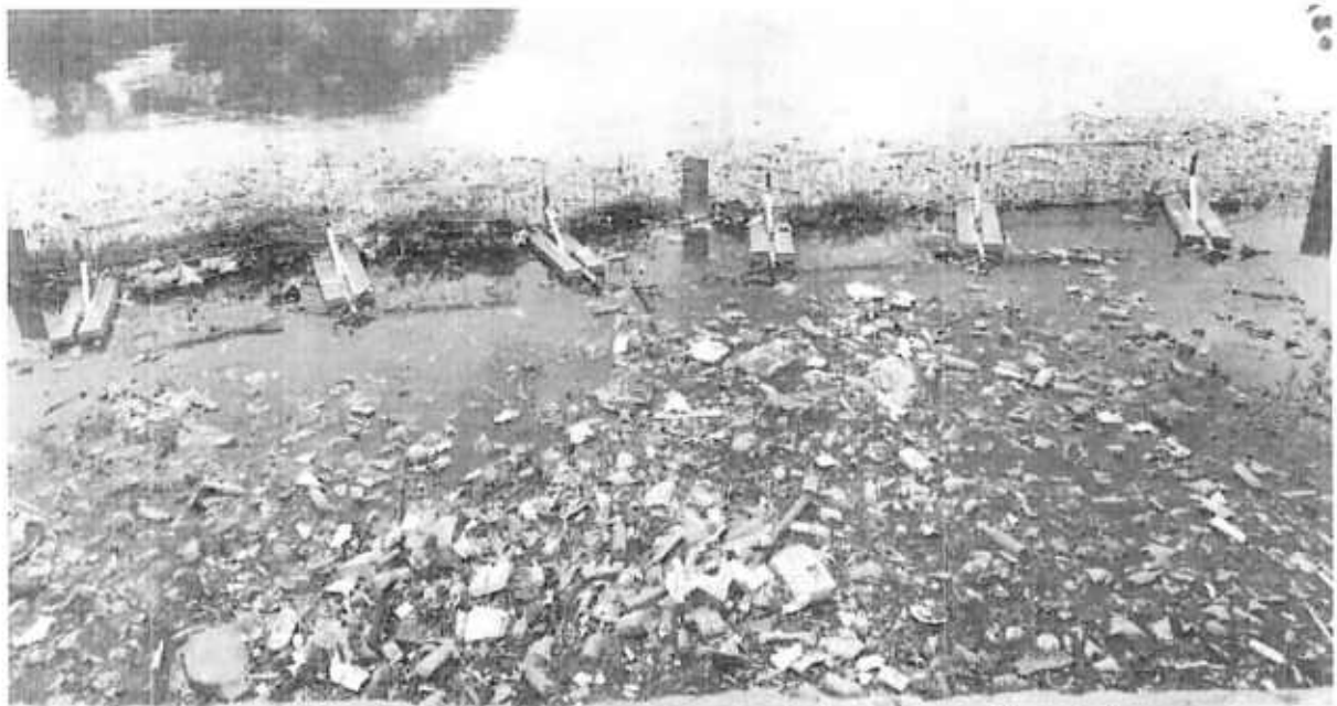
Figure 6: Debris collected at the screen installed at inlet of Ulsoor Lake
