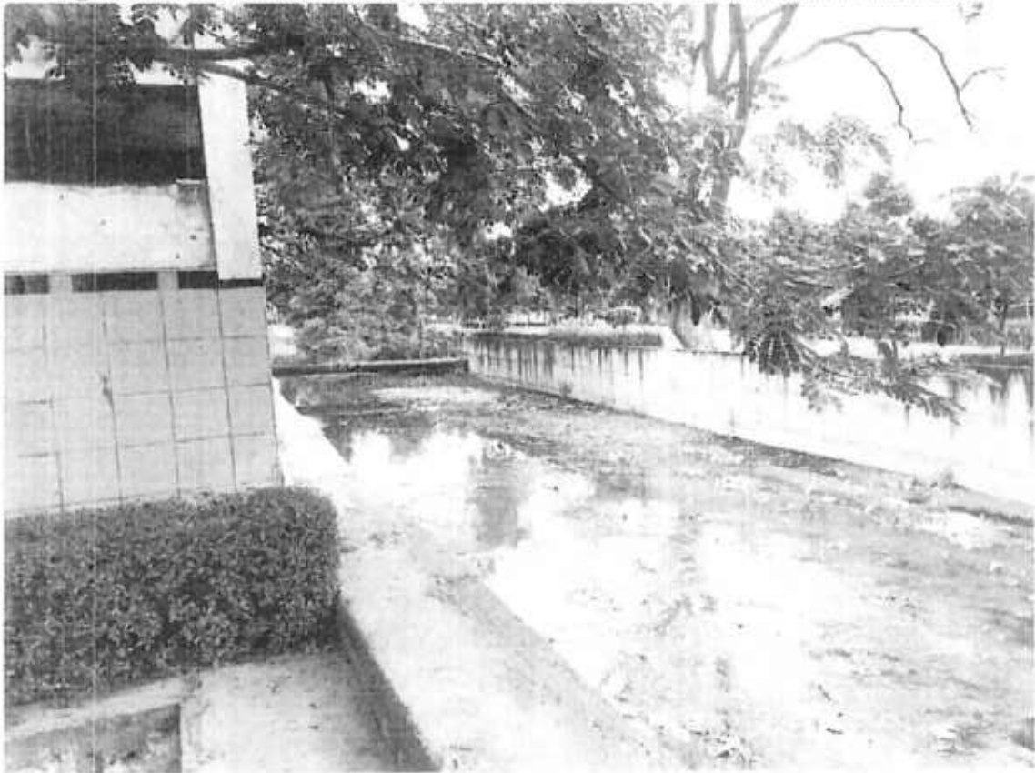
Figure 2: Flow at storm water drain C-100 downstream of Ulsoor Lake
