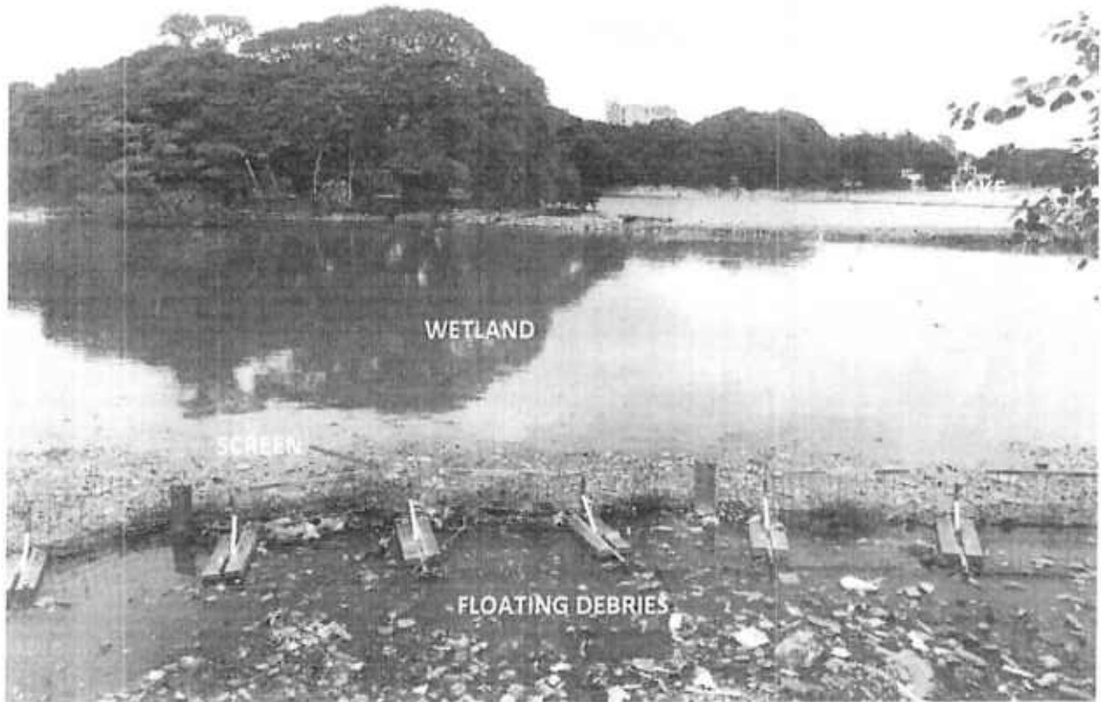
Figure 5: Screen installed by BBMP at inlet of wetland in Ulsoor Lake
