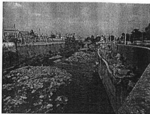
Photo.2: Telecom layout - Hosahalli main road
