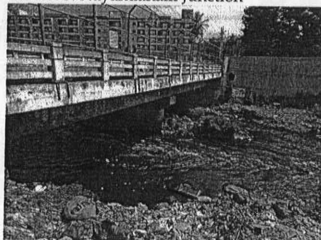
Photo.5: Nayandahalli STP D/S at RR Nagar, Temple road
