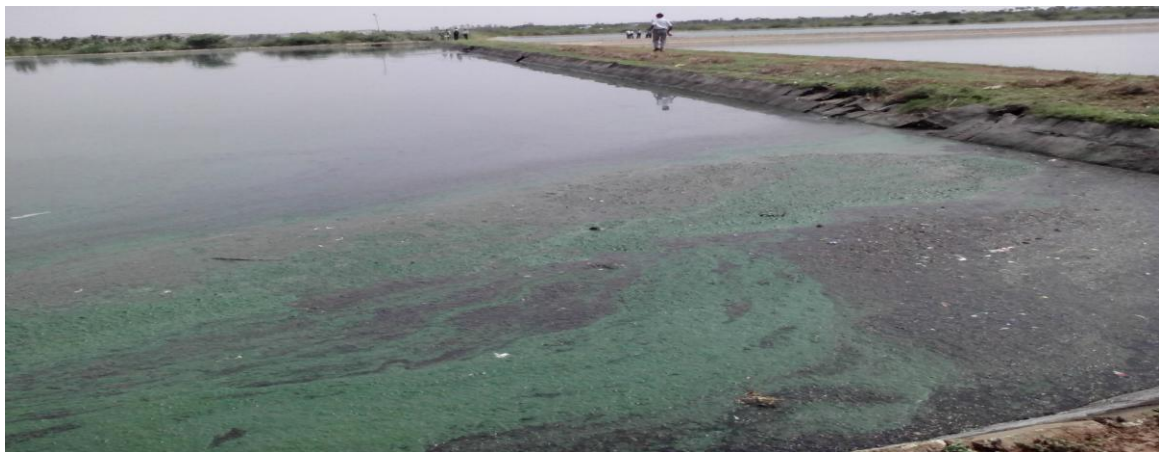
Fig 10: Facultative pond showing more algal growth on the surface
