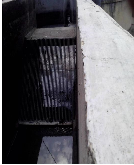
Fig 2: Screen Chamber
