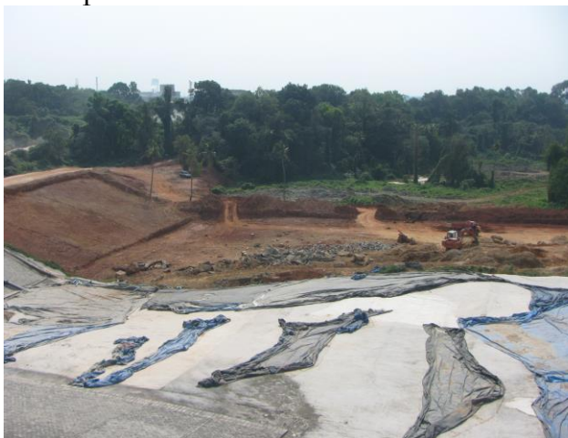
Fig.5: Cells under construction for expansion.
