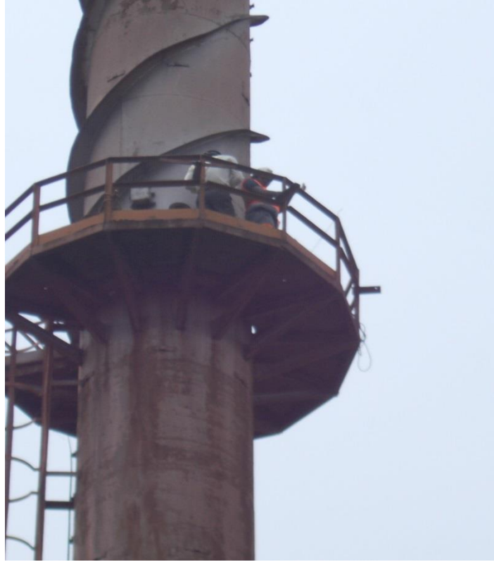
Source emission monitoring at stack attached to Sinter plant -1
