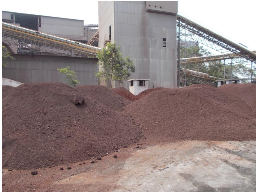
Storage of Raw material in open yard without sprinkler system to arrest the fugitive emissions
