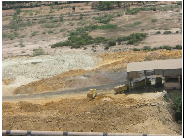
Fig.10: Sludge stored along with lime stone, charging area to the crusher
