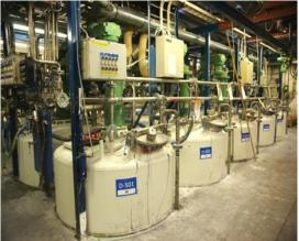
The unit representatives taken the team to their plant and shown the arrangements made for collecting VOC emissions from process and general working place and circulating system to reduce the concentration of VOC before discharging through stack.
