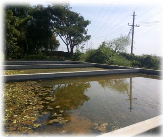
Solar Evaporation Pond
