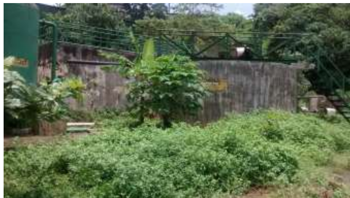
View of Treatment units
