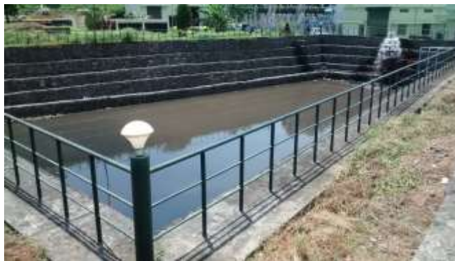
Treated Effluent Recharge Pond
