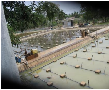
Fig 22: Solar evaporation pan
