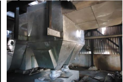
Fig 8: Dust collector
