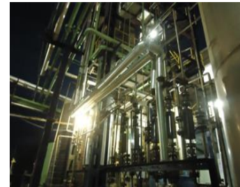
Fig 17: Double effect Evaporator
