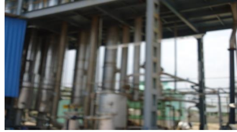
Fig 64: MEE under progress
