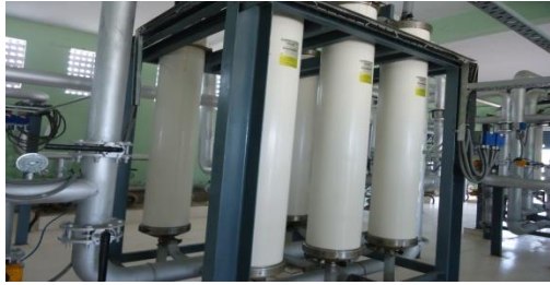
Fig 63: R.O. System under trial run
