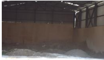
Fig 10: Hazardous waste Storage yard
