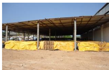
Fig. 45: Hazardous Waste storage shed (New)
