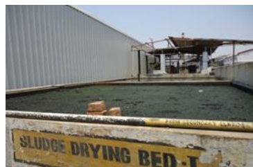
Fig 14: Sludge Drying Beds with accumulated sludge
