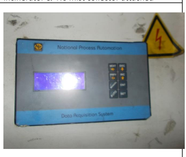
Fig.6: Process automation and data acquisition system under repair
