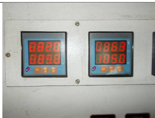
Fig.2: Operating parameter indicator, Secondary temperature showing only 863°C against 1050°C.
