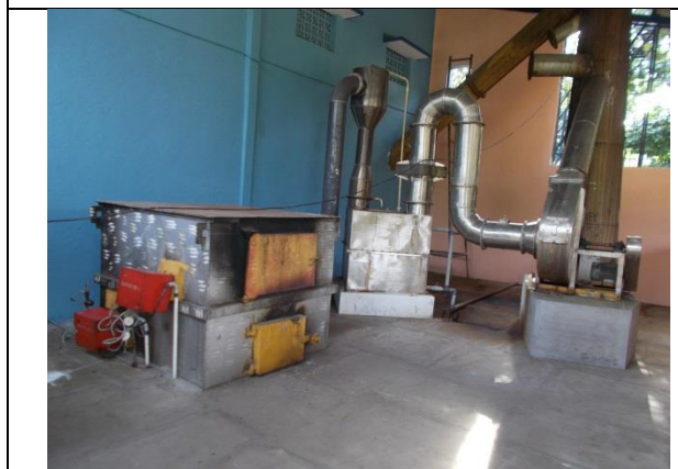
Fig.3: Incinerator of 50 kg/hr. with APCD, ID connected to common stack..
