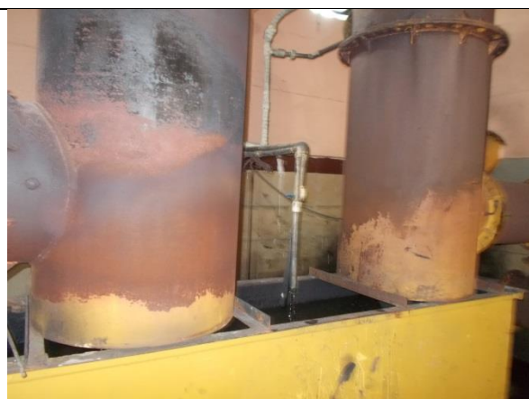
Fig.8: No pressure gauge or u- tube manometer to measure the pressure drop across the venturi
