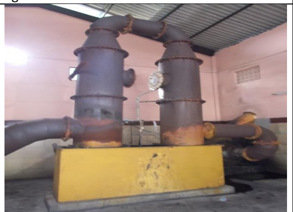
Fig.4: Scrubber connected to 100 kg/hr. incinerator & No mist collector attached
